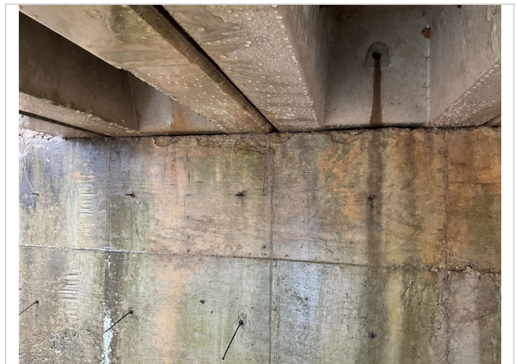
Bent 2 Minor scaling in top of abutment
